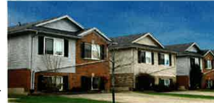
In 2004, MennoHomes completed its first project of 16 homes on Village Road in Kitchener.
